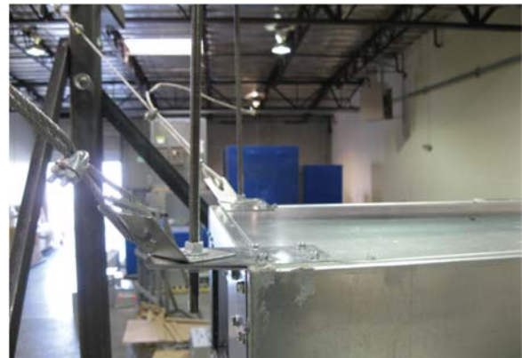
FIGURE 5 – OVERLAPPED FLAT, 90° AND 45° BRACKETS.
