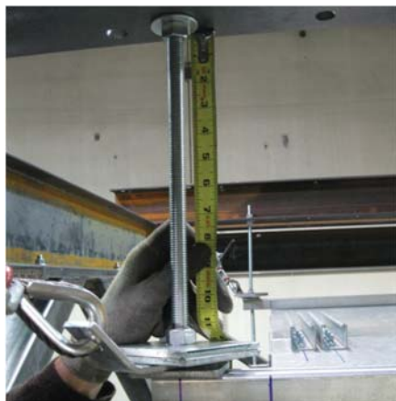
FIGURE 4 – RECOMMENDED LENGTH OF THREADED ROD
